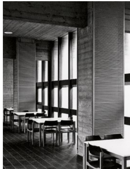
Single-column radiator as a pillar cladding around 1970. The single-column combined the modern, timeless form in an advantageous way with a low overall depth.
