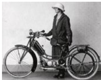
Lina Dreier from Graenichen, the sister-in-law of Arnold Zehnder, poses behind a 110 cc ladies' model. Like all early "Zehnder", the motorcycle is still equipped with a carbide lamp.
