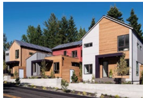
The 130 houses of the visionary "Grow Community" near Seattle, USA, are completely equipped with ventilation systems from Zehnder.
